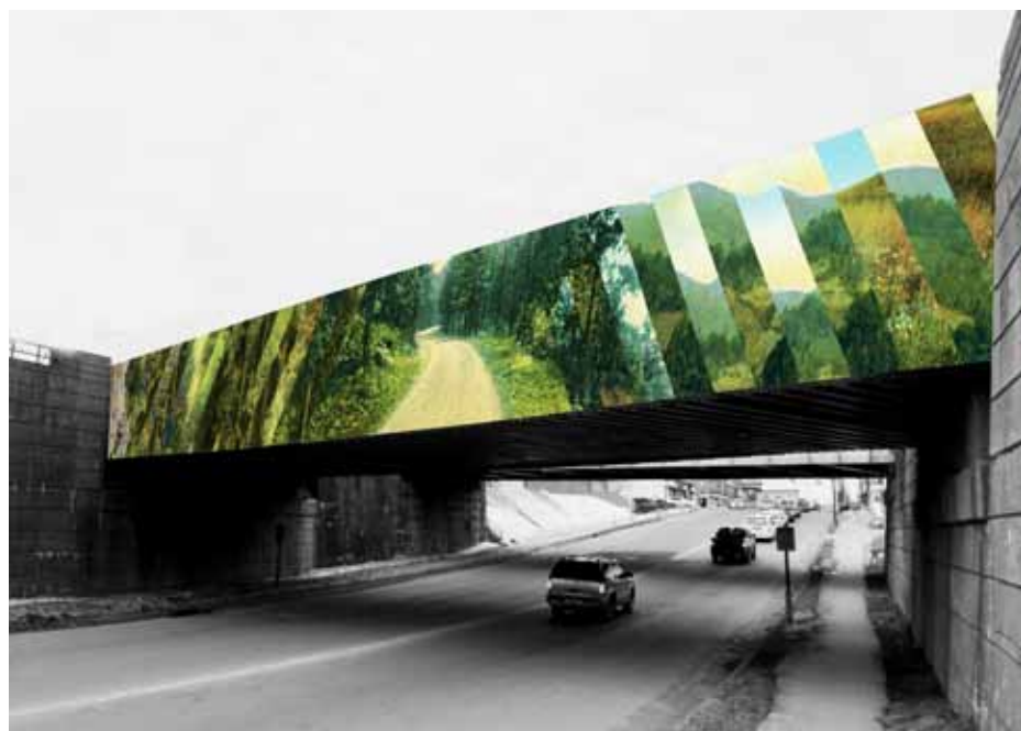
Artbridge: Kingston, a curated public art installation in Kingston, NY featuring original works by emerging Hudson Valley artists
