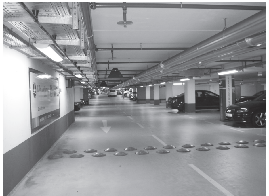
The Parking Garage below the promenade in Cologne, Germany
